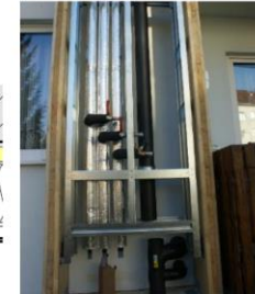
Figure 77. Installation zone (left) Section of an installation zone: (1) TES element; (2) installation zone; (3) substructure at ceiling level. Source: [1] (right) Example in London (UK)
